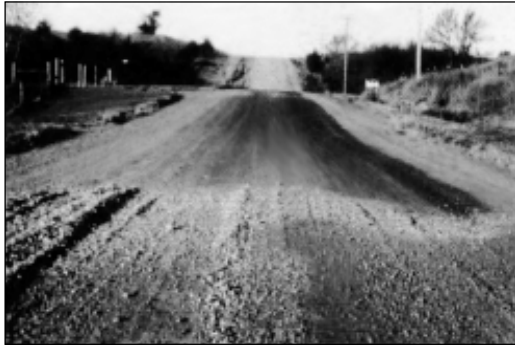
This example shows a spot treatment with magnesium chloride near a road entrance that is often a washboard troublespot.
