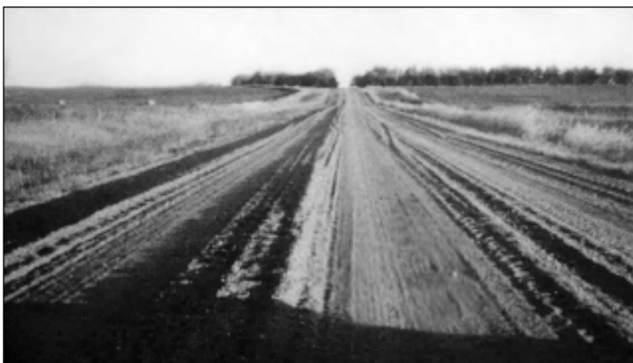
These two contrasting examples appear quite different, but the real difference is only in the surface gravel. The material on the right has a nice bleed of stone, sand and fines which remain tightly bound and resist washboarding.
