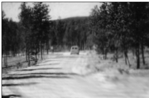
No washboarding is evident, even on the curve of this road, which is surfaced with good quality gravel and treated with magnesium chloride.
