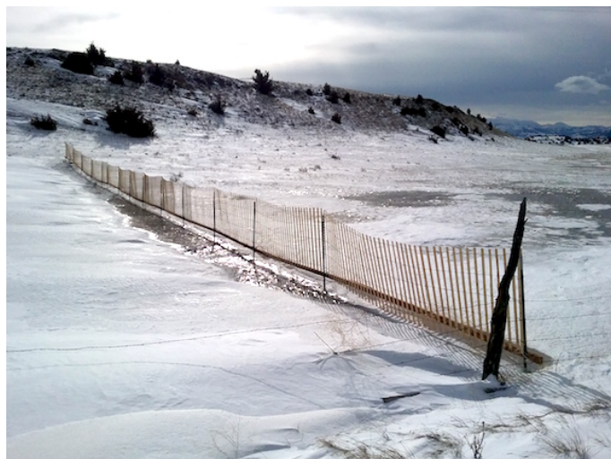
Above: Snow fence with new design that raises the fence 12 inches above ground resting on pressure-treated 2' x 4's.
