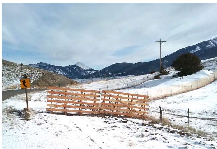
Above: The horizontal snow barrier at the top of Sirius Hill.
